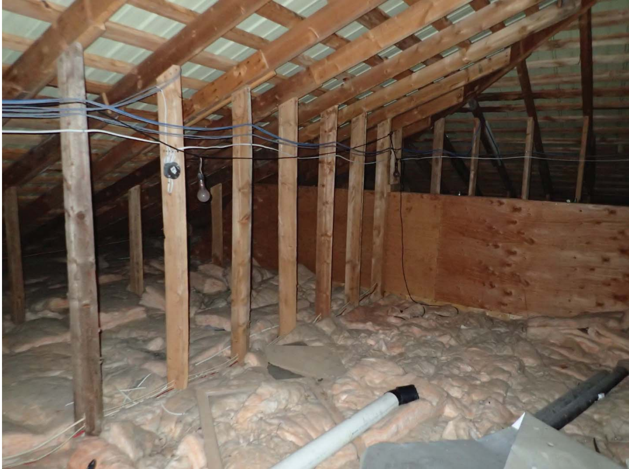
Photo 3: Struts supporting the roof rafters.
