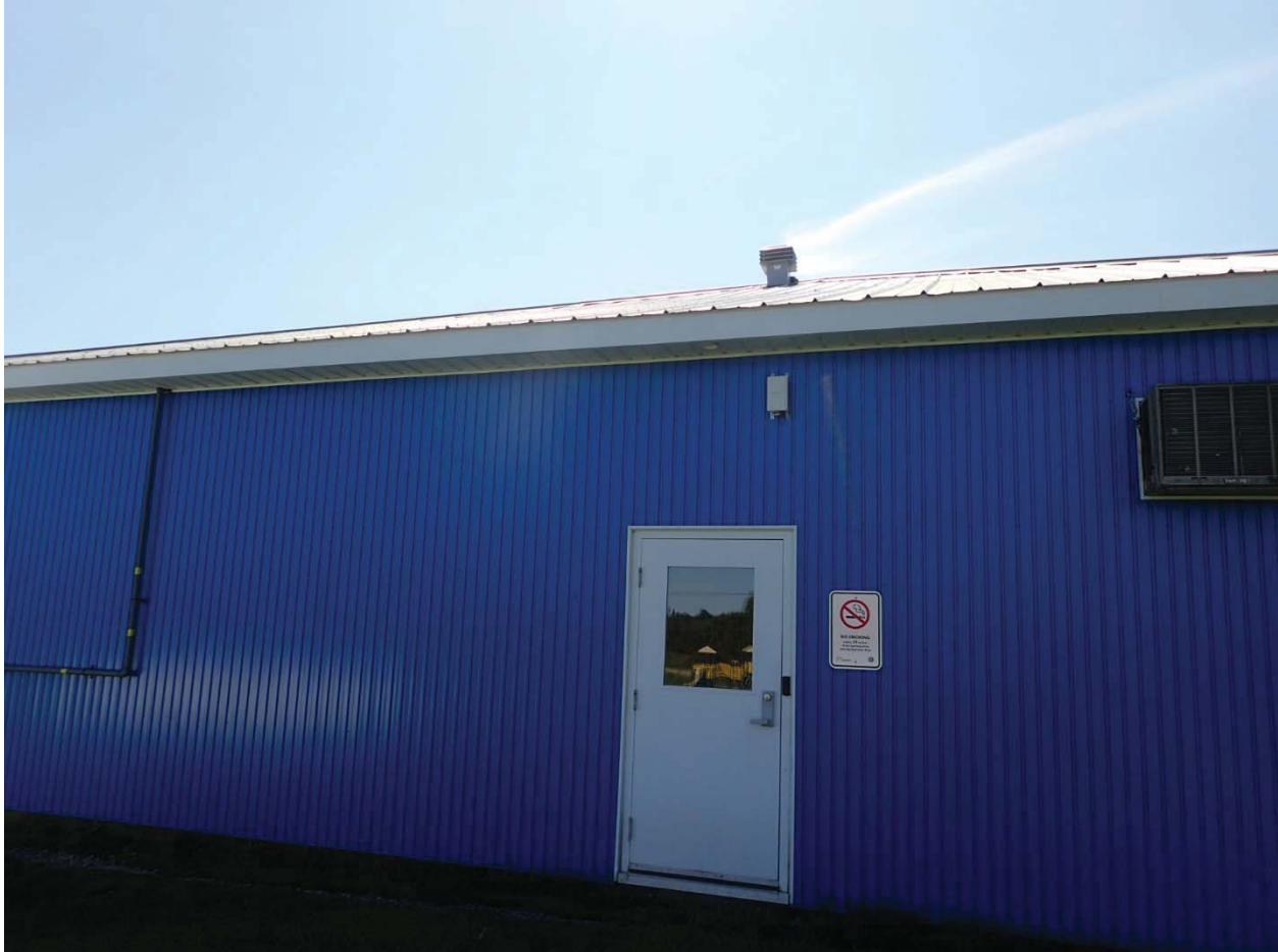
Photo 7: The north face of the building.
