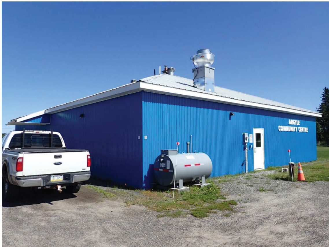
Photo 1: View of the front of the community centre.
